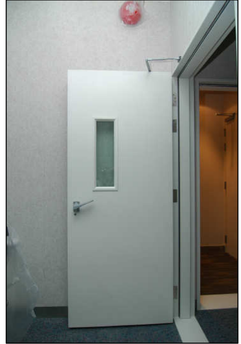
Acoustic Glass Vision Panel Design
